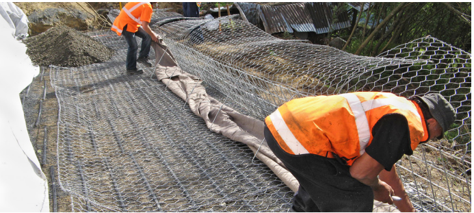
Fig. 12 – Placing erosion control blanket
