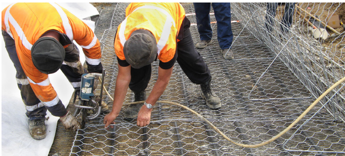
Fig. 9 – Connecting adjacent units with rings
