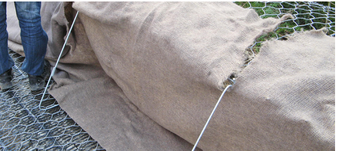
Fig. 13 – Slitting erosion control blanket
