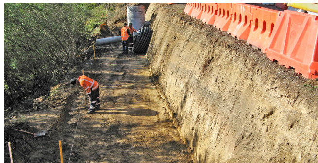
Fig. 5 – Prepared foundation
