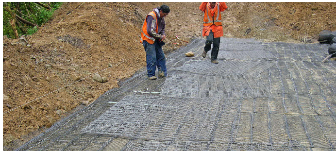
Fig. 7 – Placing units in position
