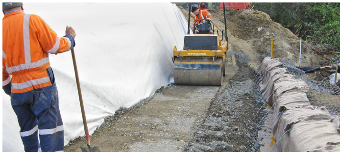
Fig. 14 – Compaction of structural fill
