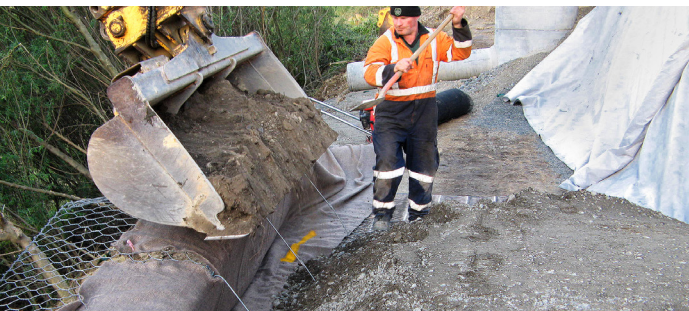
Fig. 15 – Topsoil placement
