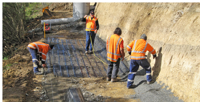
Fig. 6 – Placing geogrid
