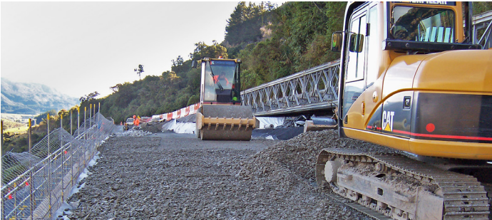
Fig. 14 – Fill placement and compaction
