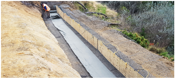
Fig. 13 – Laying out nonwoven geotextile
