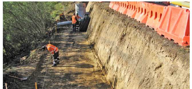
Fig. 5 – Prepared foundation
