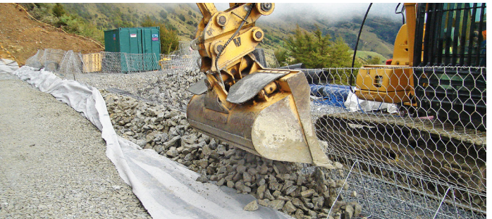
Fig. 16 – Rock placement
