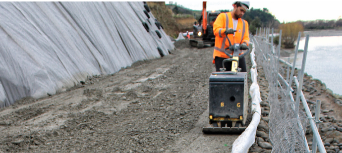
Fig. 15 – Compaction close to the face
