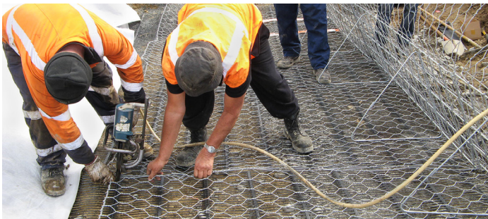
Fig. 9 – Connecting adjacent units with rings
