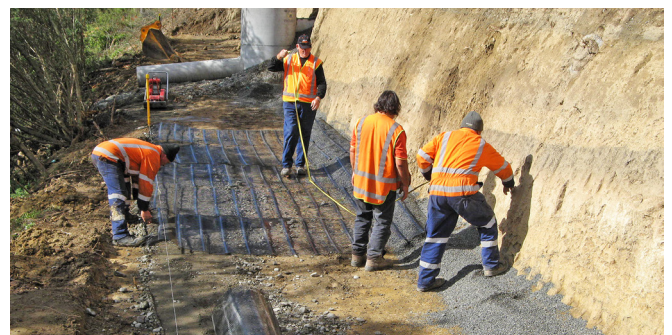
Fig. 6 – Placing geogrid
