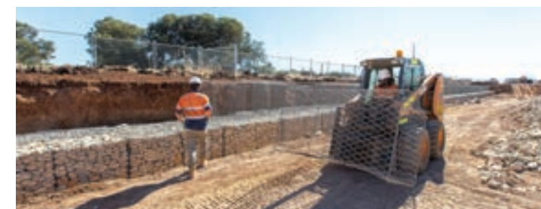
Fig. 12 - Gabion layout to allow for an easier installation
